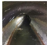
(B) Culverted stream CC00183 at inlet facing downstream
